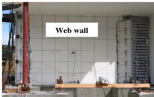
Figure 13. State of damage for EQ4 test
