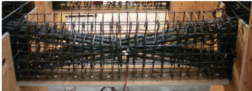
(a) Coupling beam with reinforcement congestion
