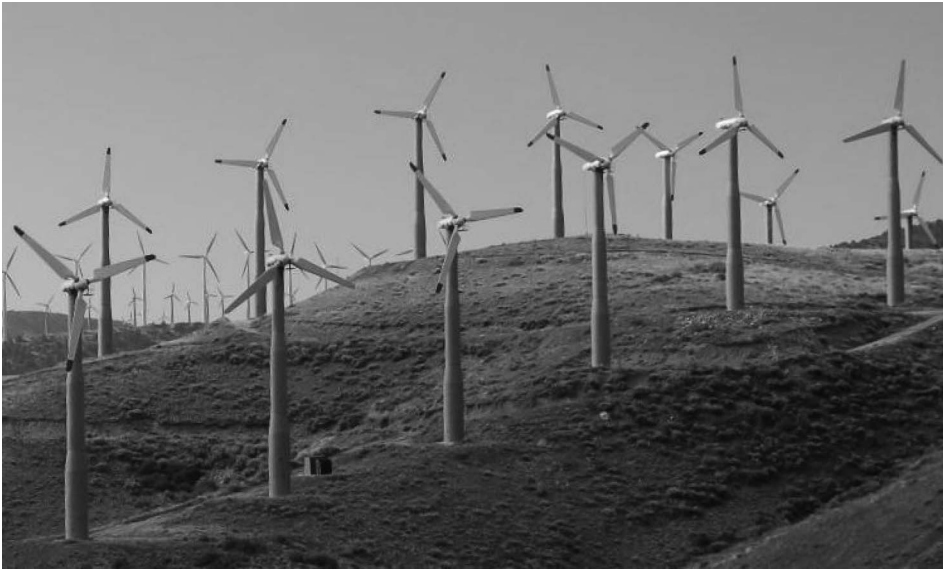
FIGURE 3 Field installation at Oak Creek Energy Systems in Tehachapi, CA.
